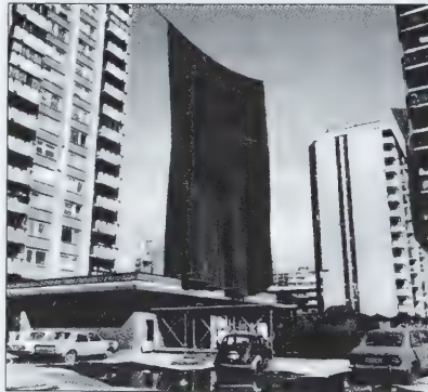
Hrasno, the Sarajevo Community which has linked to Amsterdam, is dominated by high-rise blocks of flats, badly damaged by shelling. A question now confronting the Community is whether to restore this housing or demolish it and start afresh.
