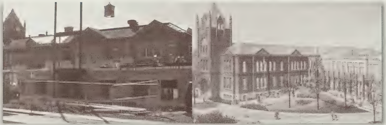
(l) Goodes Hall construction site from Albert Street, September 2001
