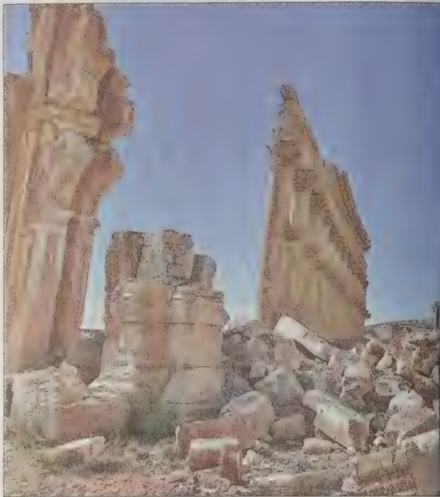
Damage inflicted by Islamic State militants is seen in the ancient city of Palmyra, Syria.
