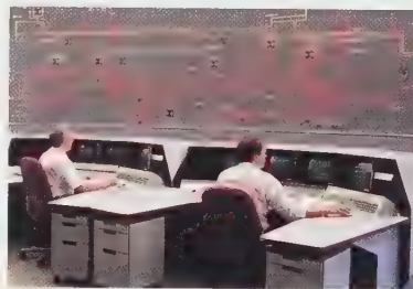
The Data Acquisition and Computer System (DACS) gathers status information from all Ontario Hydro generating, transformer and switching stations.
