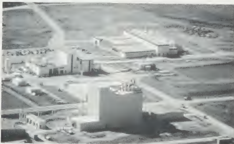
The Aldrich plant at Sheboygan, WI. (There is no picture of the garage in Milwaukee where the company started its operations.)
