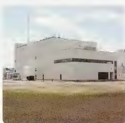
Pro I building at Aldrich's Sheboygan County site.
