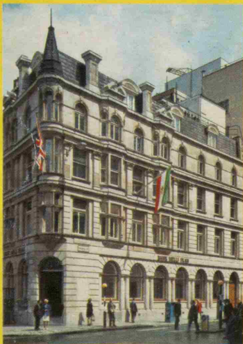
Premises of London Branch at Leadenhall Street
