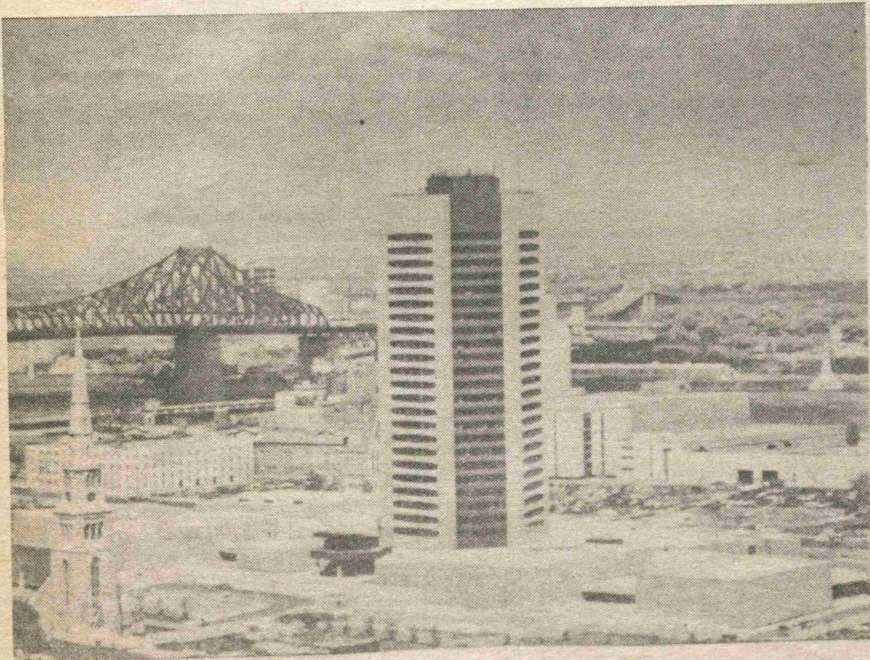
Looking south-east from the centre of Montreal, the Maison Radio-Canada is shown with the Jacques Cartier Bridge spanning the St. Lawrence River in the background
