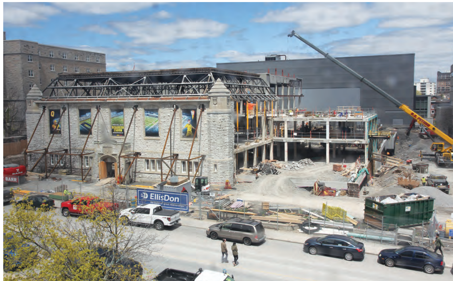
The new Innovation and Wellness Centre will include the original limestone façade. Queen's will also reinstate the original windows.
